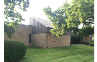
Existing Warren Branch Library
